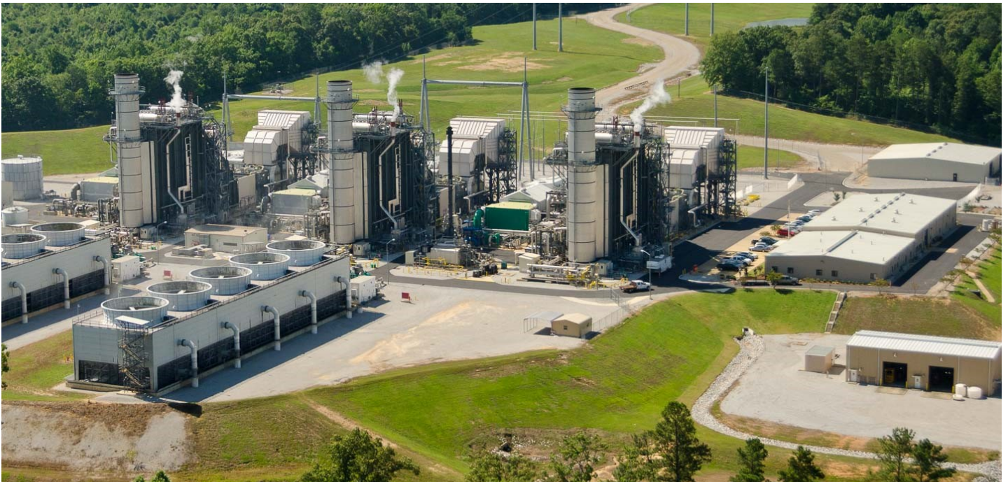
Natural Gas Power Plant
