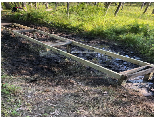
Frame under the new boardwalk. See article on page 14 (digital version)
